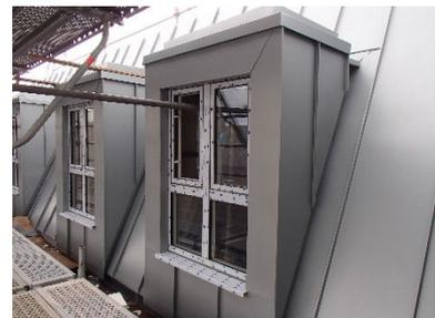
The roof over the apartments has been insulated and sealed with the weatherproof layer of single ply membrane. The rendered finish is now being applied to the section next to Costa. Here the windows have a feature surround and the walls incorporate ashlar grooves and band courses. The completion of these finishes releases the scaffolding. Therefore during this month you will see the scaffolding being progressively dismantled and the hoarding removed to allow works to commence on the pavements.
