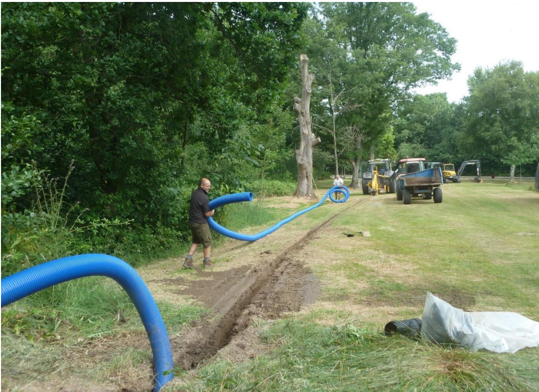
Laying the pipe in the main drain.
